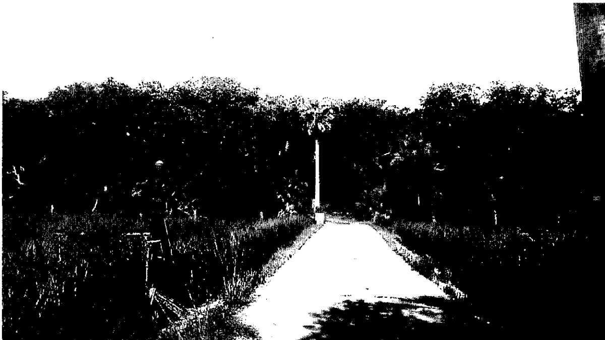
Figure 1. Subject property viewed looking southeast toward Island 11 showing notice sign posted and condition of causeway.
